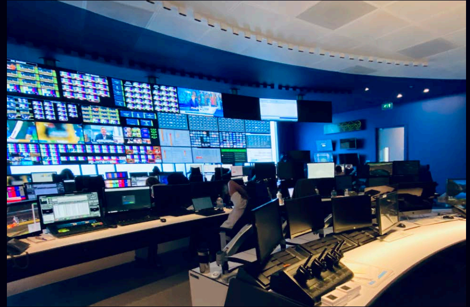
Encompass Control Room, London
